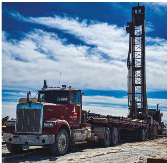
Drilling of Jackson-31 well
