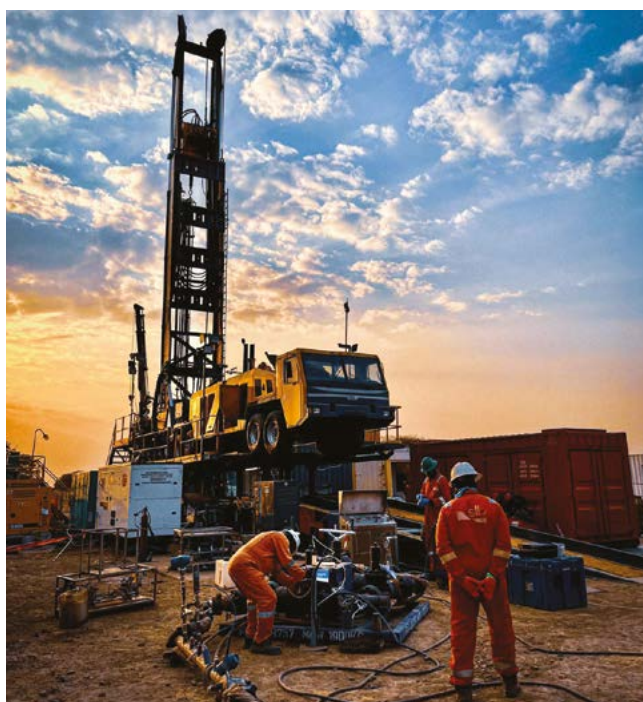
ITW-1 well test
