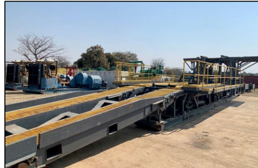
Assembly of rig substructure Tai-C well site
