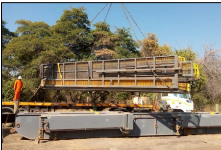
Equipment arriving at Rukwa lay down area
