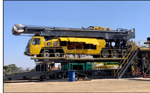
Rig raised on substructure Tai-C
