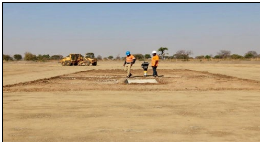
Completion of Tai-C well site and concrete pad
