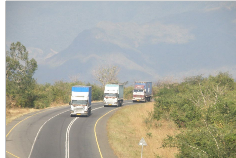
TanZam Highway, 920km hard top road linking site to Dar es Salaam Port
