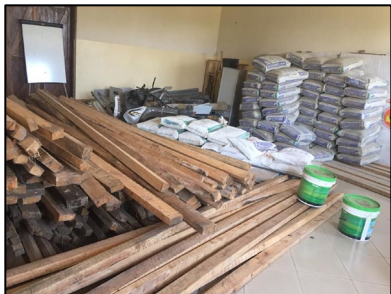
Building materials supplied by He1
