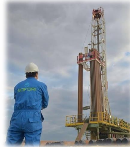
SOFORI Rig Drillmec HH102 – on location in Tunisia
