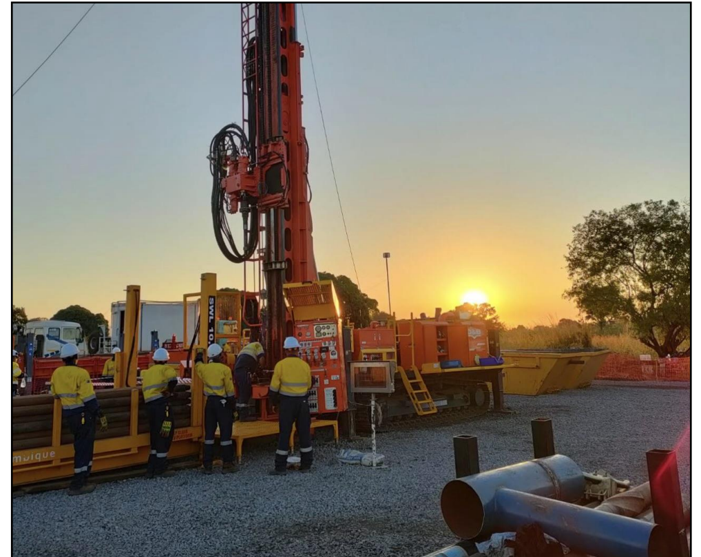
Mitchell Drilling rig at Tai-1/-1A (2021)
